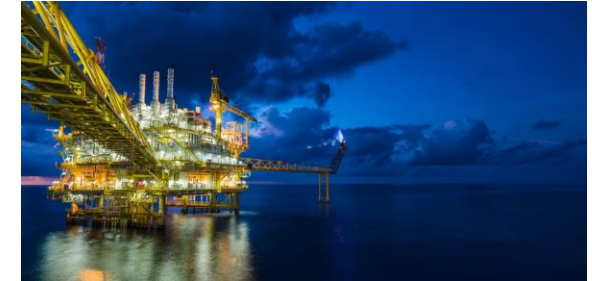
Oil and gas central processing platform. © Shutterstock
