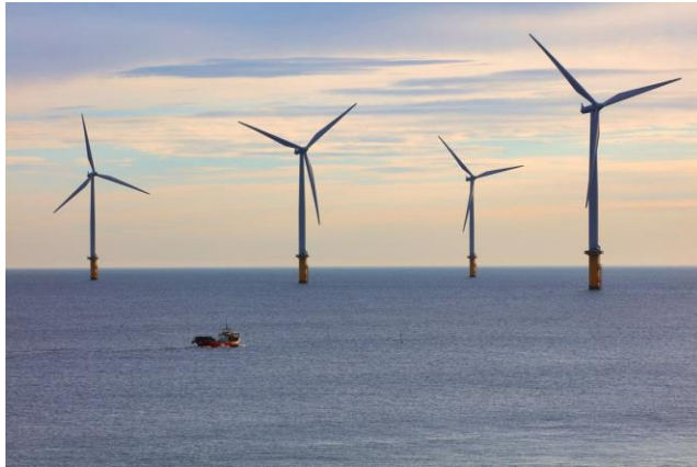
Offshore wind turbines off the North-East Coast of the United Kingdom. © Colin Ward
