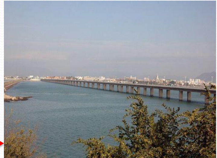
The cross-sea bridge in Xiamen
