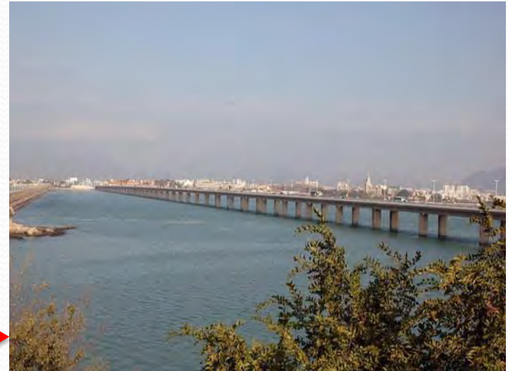
The cross-sea bridge in Xiamen
