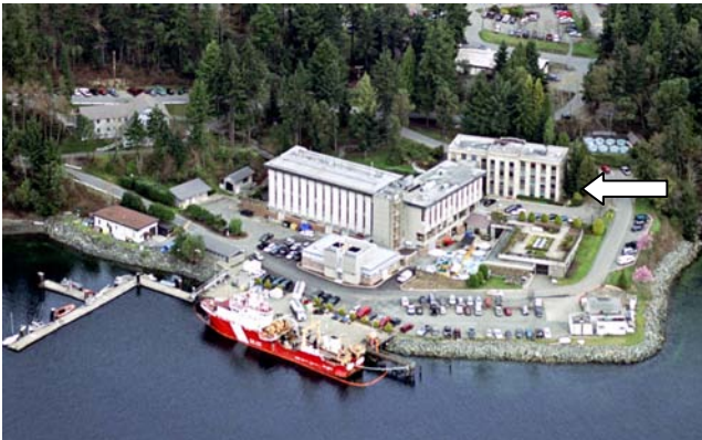
Pacific Biological Station (PBS) in 1912 (above) and 2008 (below). The original structure was demolished to accommodate in 1948 what is now known as the Clemens Wing (arrow inset).
