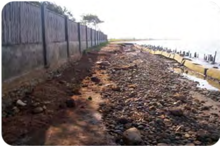
Coastal Erosion in Pekalongan
