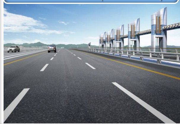
4-lane road (Left Side)
