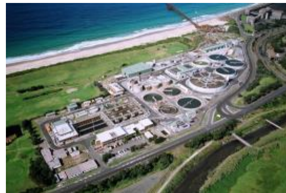
Sewage plant (NSW)
