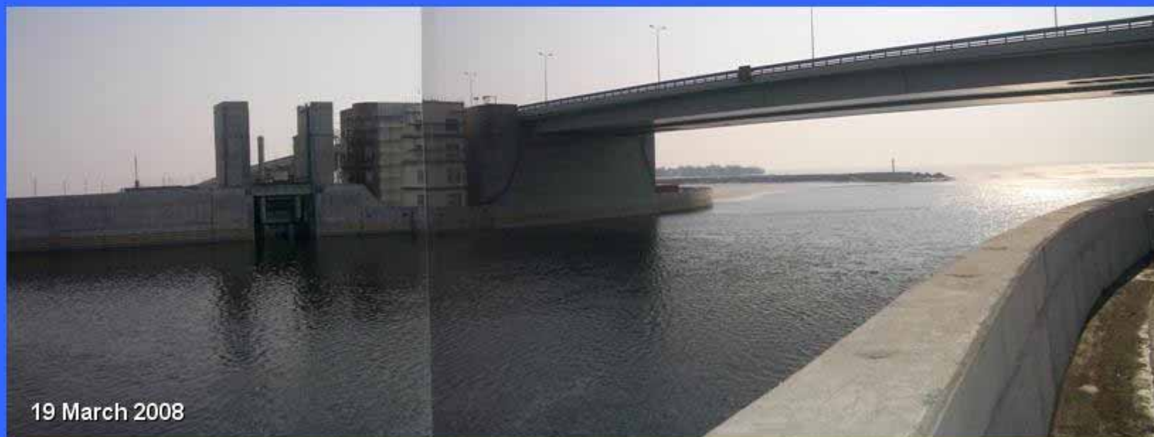
Navigation sluice C-2 for local ships is almost completed
