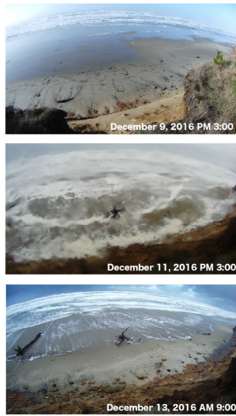
Fig. 4| Photographs of the day before (December 9, 2016), during which (December 11), and after (December 13) the westerly winds prevailed at the spring tide. The change of the ground form just below the webcam resulted from the landslide occurred due to the storm on December 11.
